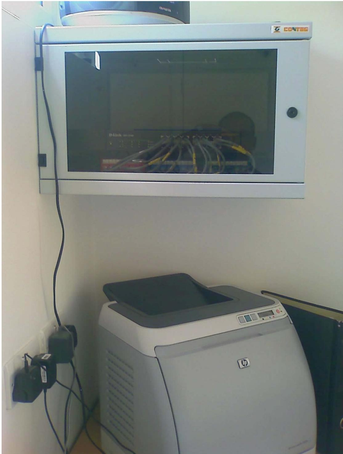
All connections were tested and certified to CAT5E standards and the link circuit to the house was completed. The alarm unit was fitted and tested with end user training given.
