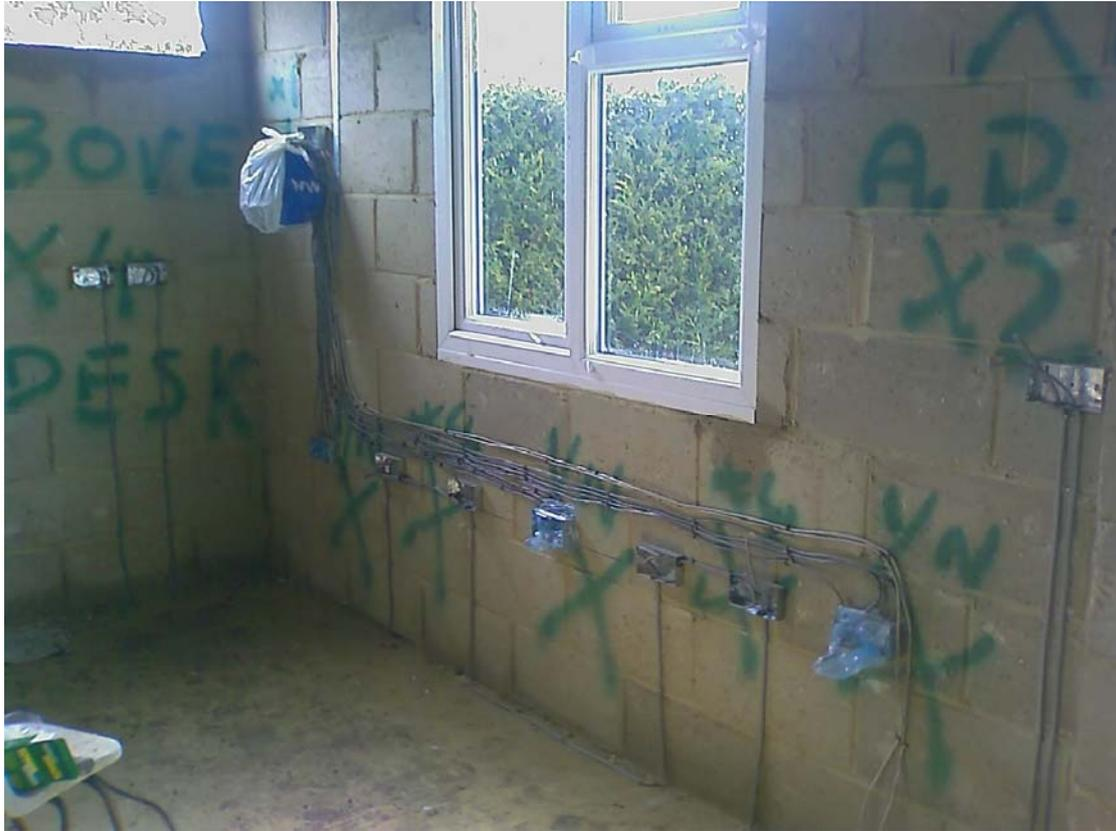
The builders then finished the walls with thermaboard to a depth of 27mm and we returned to complete the final fit. The network boxes were fitted to the walls and the IDC inserts wired up and tested.
