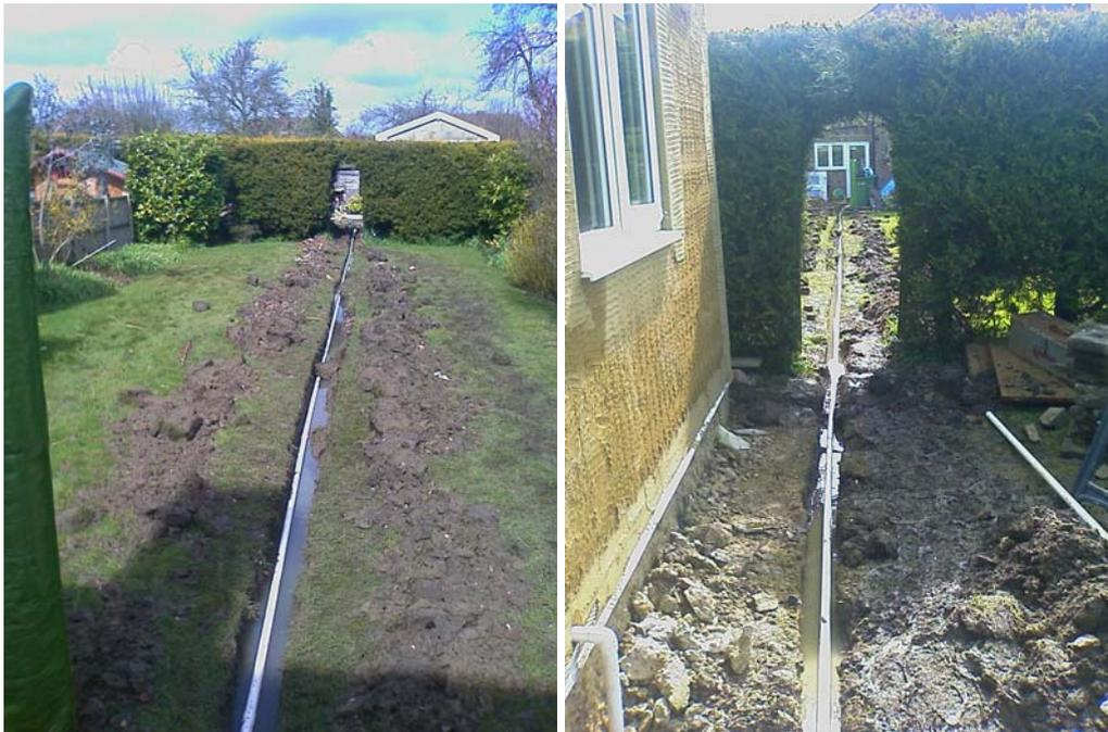
The pipes are solvent welded and watertight, running to the front of the house.
